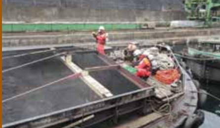
Gas detection work on fire ships
