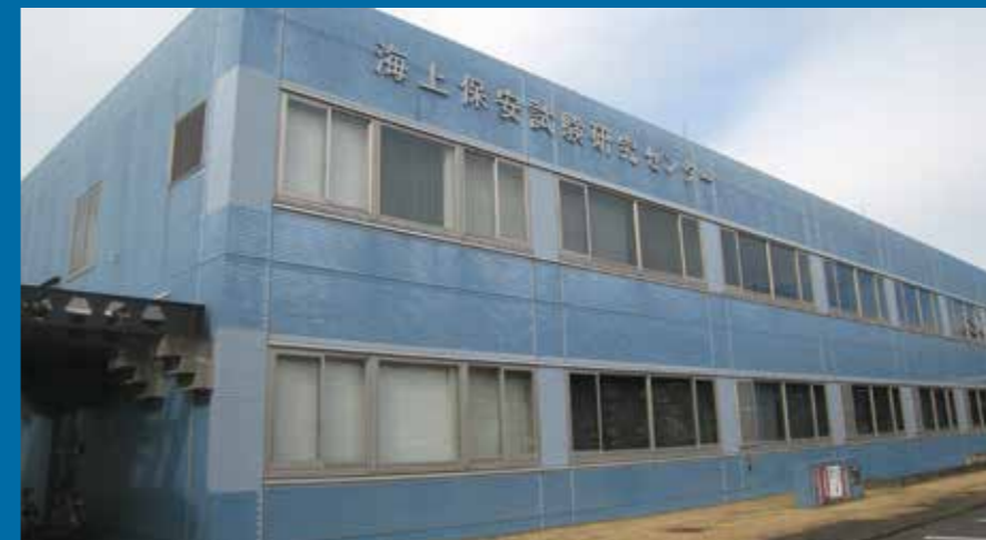
Located in the Tachikawa Regional Disaster Management Base (Tachikawa City, Tokyo), the Center can serve as the JCG's anti-disaster headquarter while the JCG's Central Government building has been hit by a disaster.
