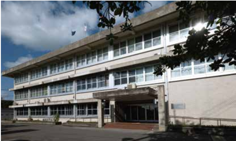
Port and harbor Joint Government Building
